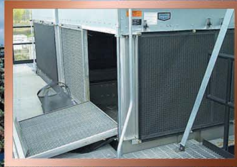
Cooling Equipment Air Intakes Portable Chillers And 125 Ton Cooling Tower
