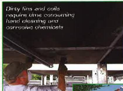
Dirty fins and coils require time consuming hand cleaning and corrosive chemicals
