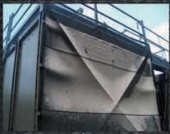
Willoworeek Church Marley Cooling Tower
